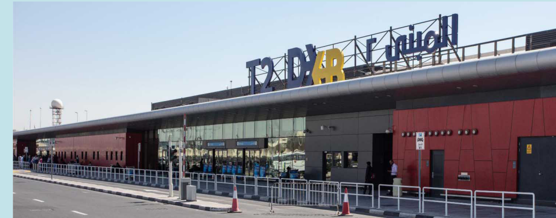
© DUBAIRPORTS. Terminal 2 Dubai International Airport
